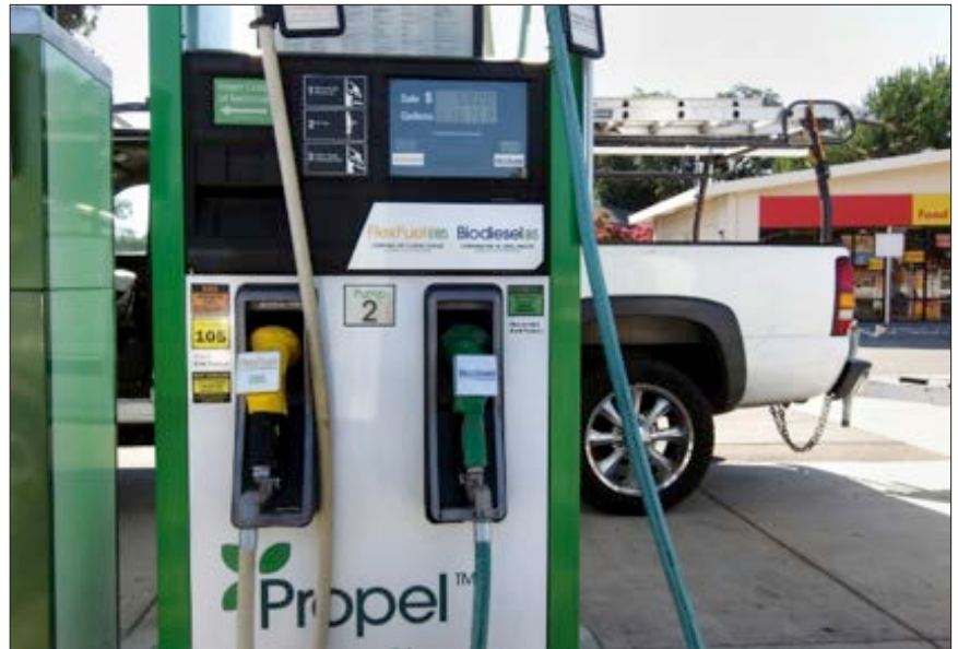
A pump that dispenses both E85 gasoline and B5 biodiesel “green” fuels. (Image: RCB, CC BY 2.0)
